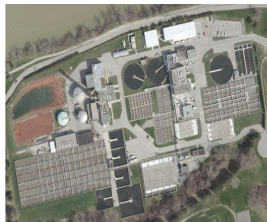
London's Greenway Wastewater Treatment Plant
